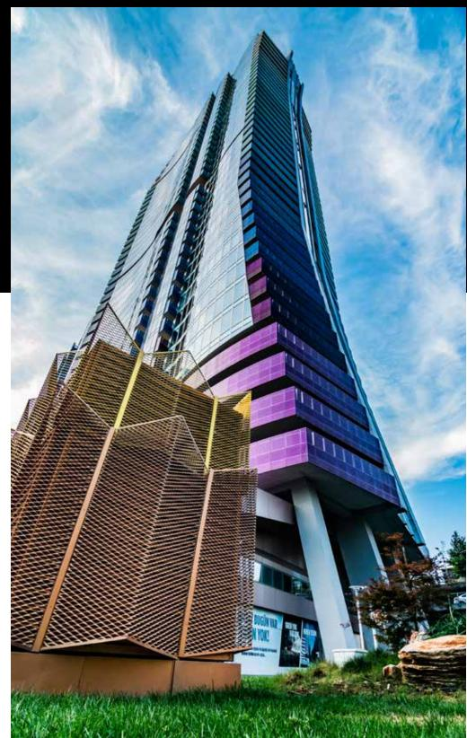
Production Date: 2016 Project Location: Maslak Materials used: Panels made of aluminum sheets and profiles were used. Areas Used: Facade
